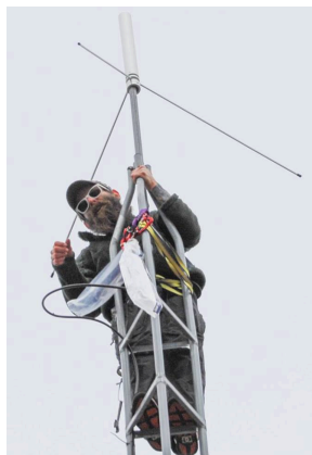
Ari atop the tower
